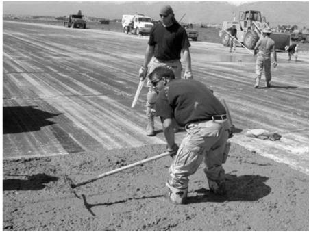
A bull float with a fixed knuckle joint may force workers to bend forward and work in awkward postures.
